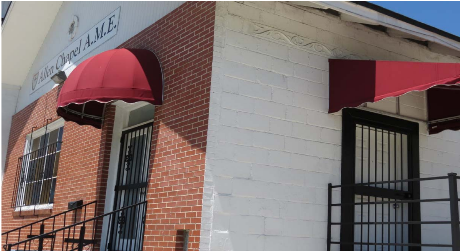
LM-19-01 ALLEN CHAPEL A.M.E. CHURCH 1529 SWAN STREET PHOTO # 19 APRIL 17, 2018
