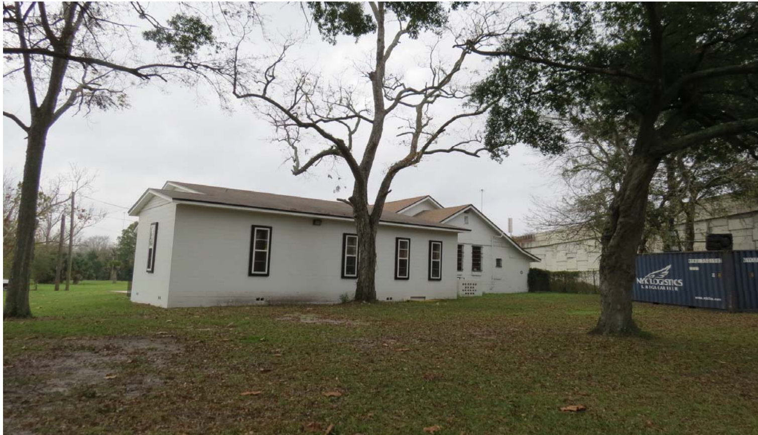
LM-19-01 ALLEN CHAPEL A.M.E. CHURCH 1529 SWAN STREET PHOTO # 9 JANUARY 4, 2019
