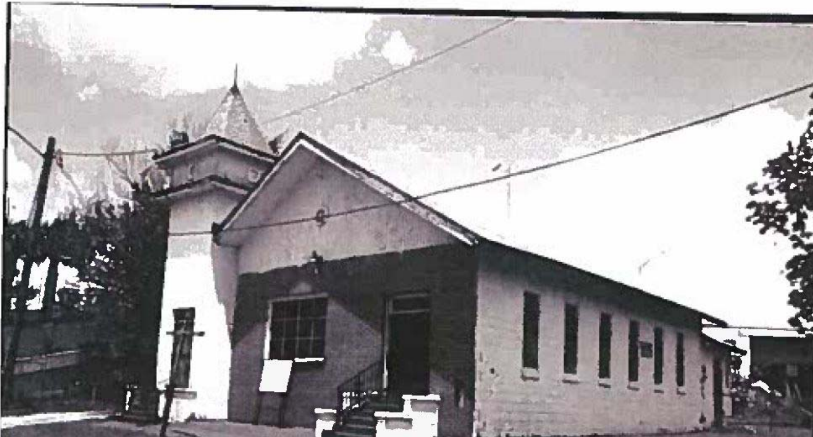
LM-19-01 ALLEN CHAPEL A.M.E. CHURCH 1529 SWAN STREET PHOTO # 7, OLDER PHOTO OF CHURCH
