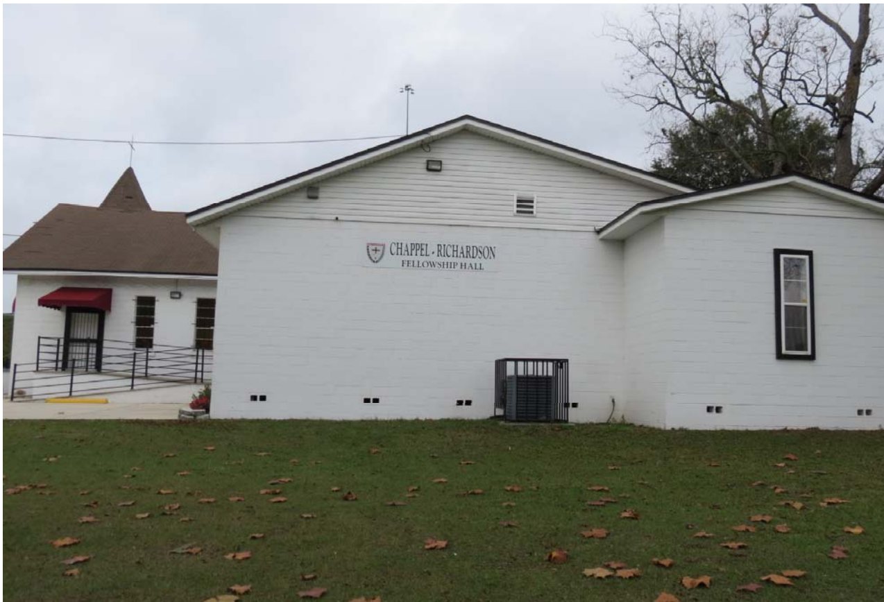
LM-19-01 ALLEN CHAPEL A.M.E. CHURCH 1529 SWAN STREET PHOTO # 27 JANUARY 4, 2019
