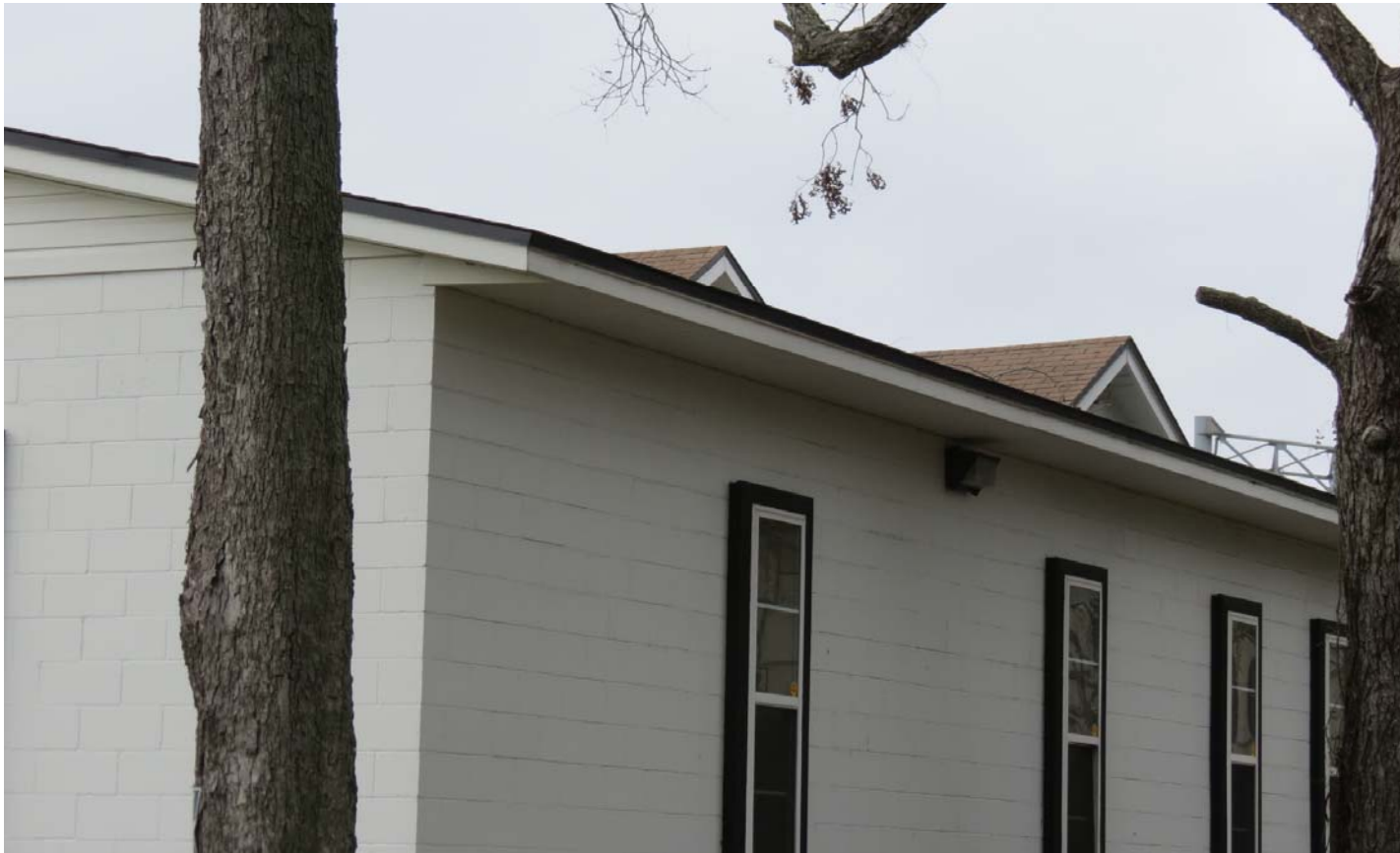
LM-19-01 ALLEN CHAPEL A.M.E. CHURCH 1529 SWAN STREET PHOTO # 36 JANUARY 4, 2019
