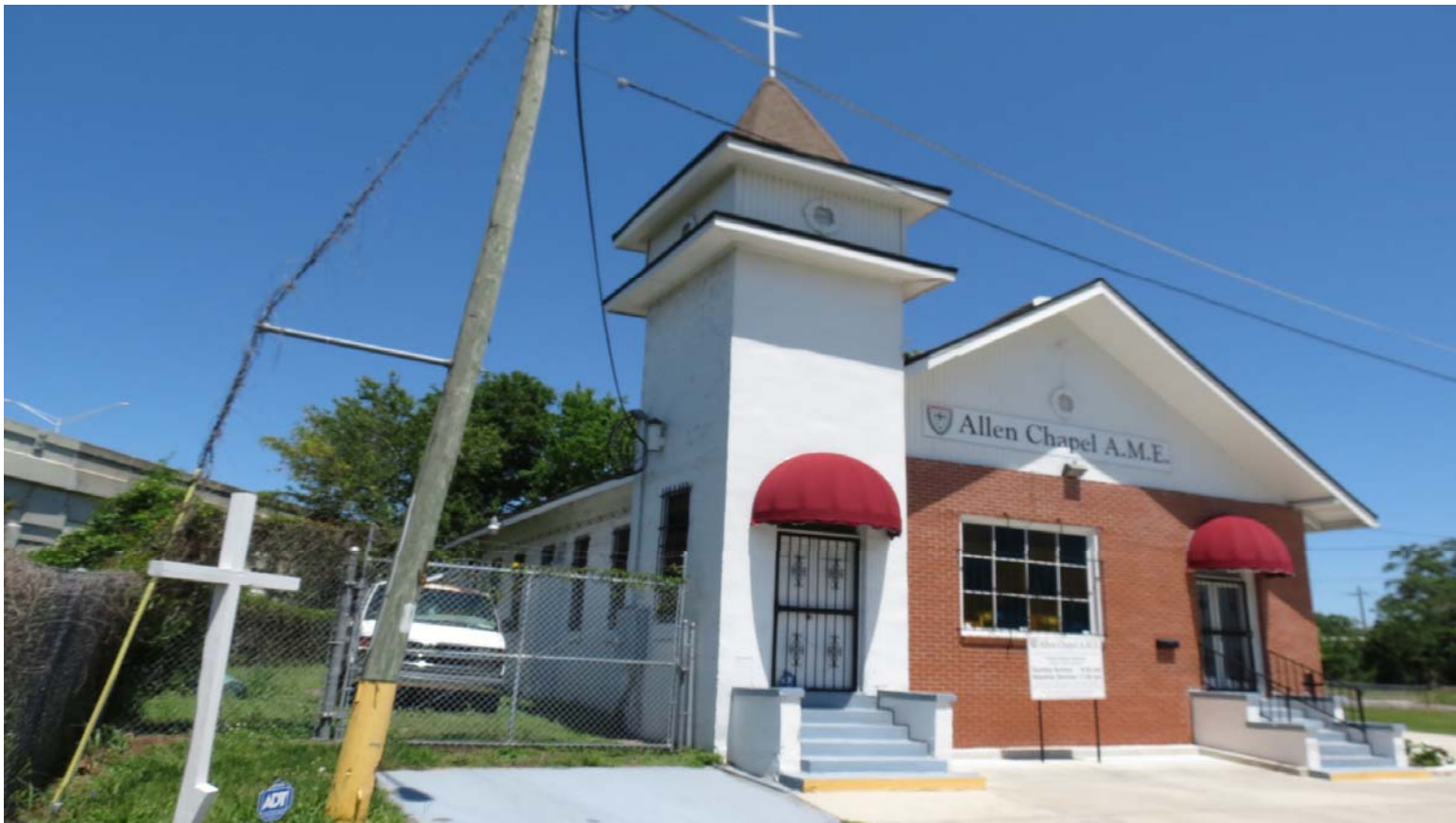
LM-19-01 ALLEN CHAPEL A.M.E. CHURCH 1529 SWAN STREET PHOTO # 17 APRIL 17, 2018
