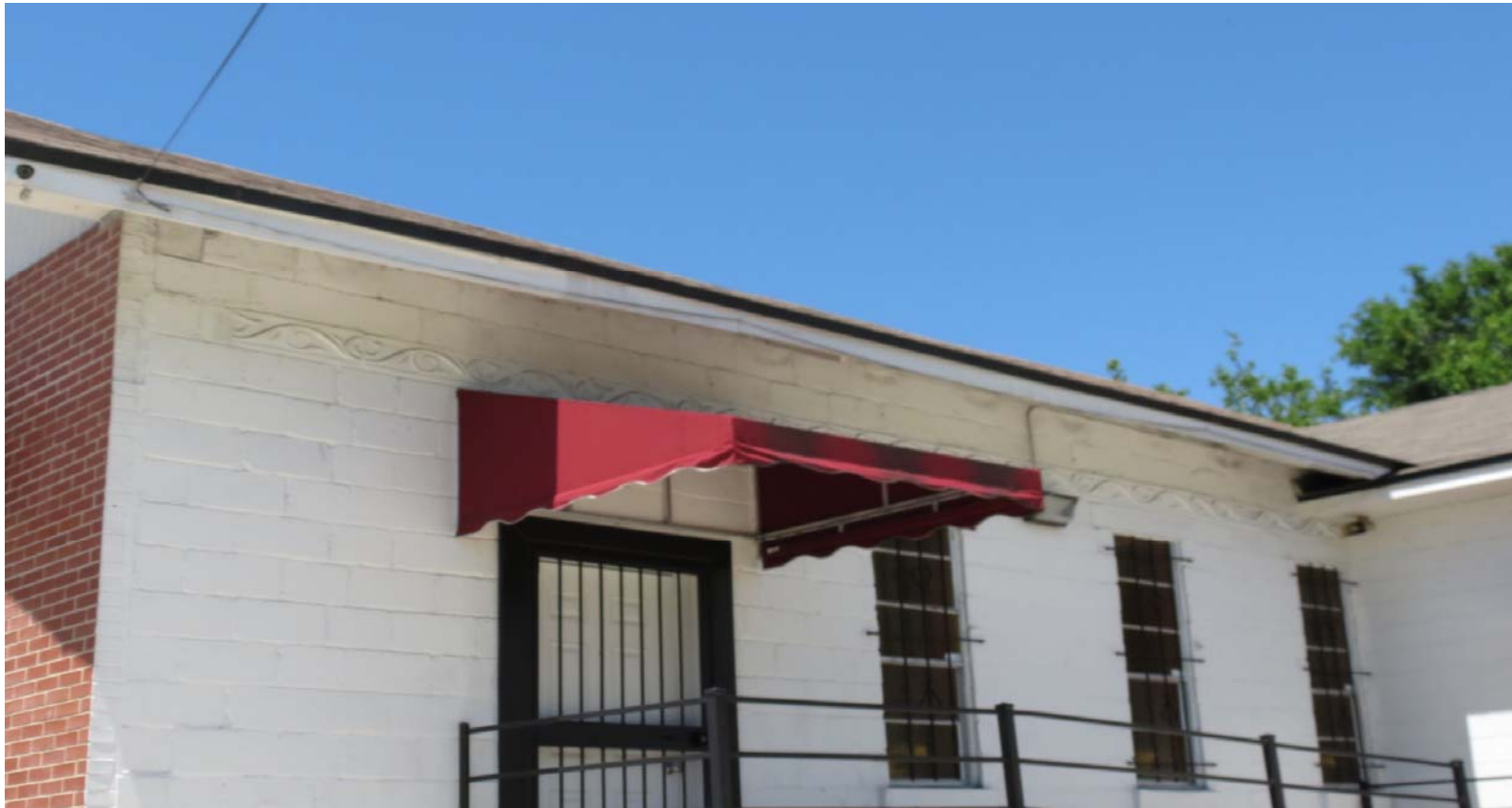
LM-19-01 ALLEN CHAPEL A.M.E. CHURCH 1529 SWAN STREET PHOTO # 24 APRIL 17, 2018
