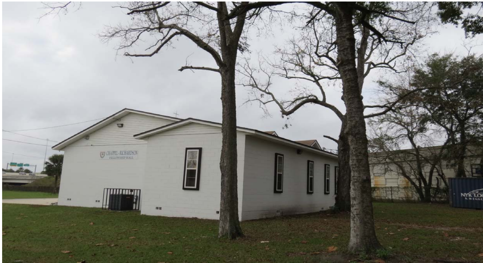
LM-19-01 ALLEN CHAPEL A.M.E. CHURCH 1529 SWAN STREET PHOTO # 35 JANUARY 4, 2019
