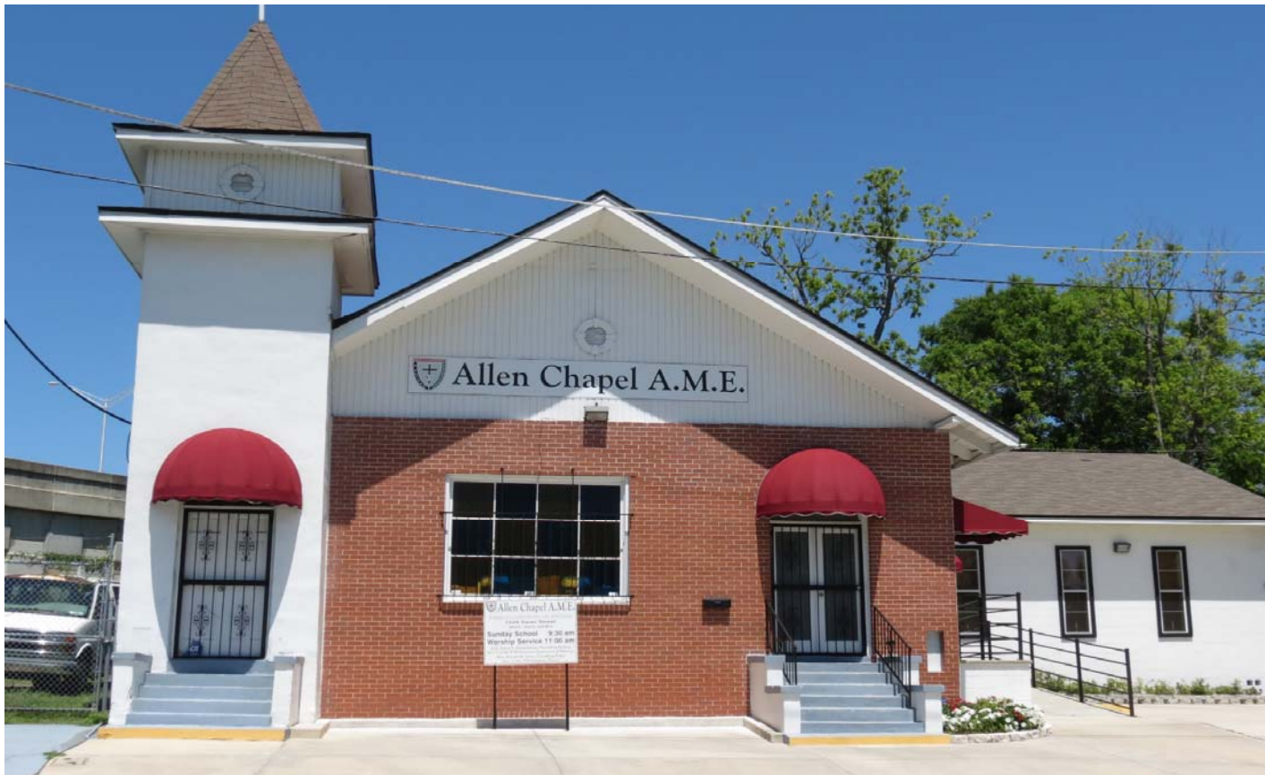
LM-19-01 ALLEN CHAPEL A.M.E. CHURCH 1529 SWAN STREET PHOTO # 16 APRIL 17, 2018
