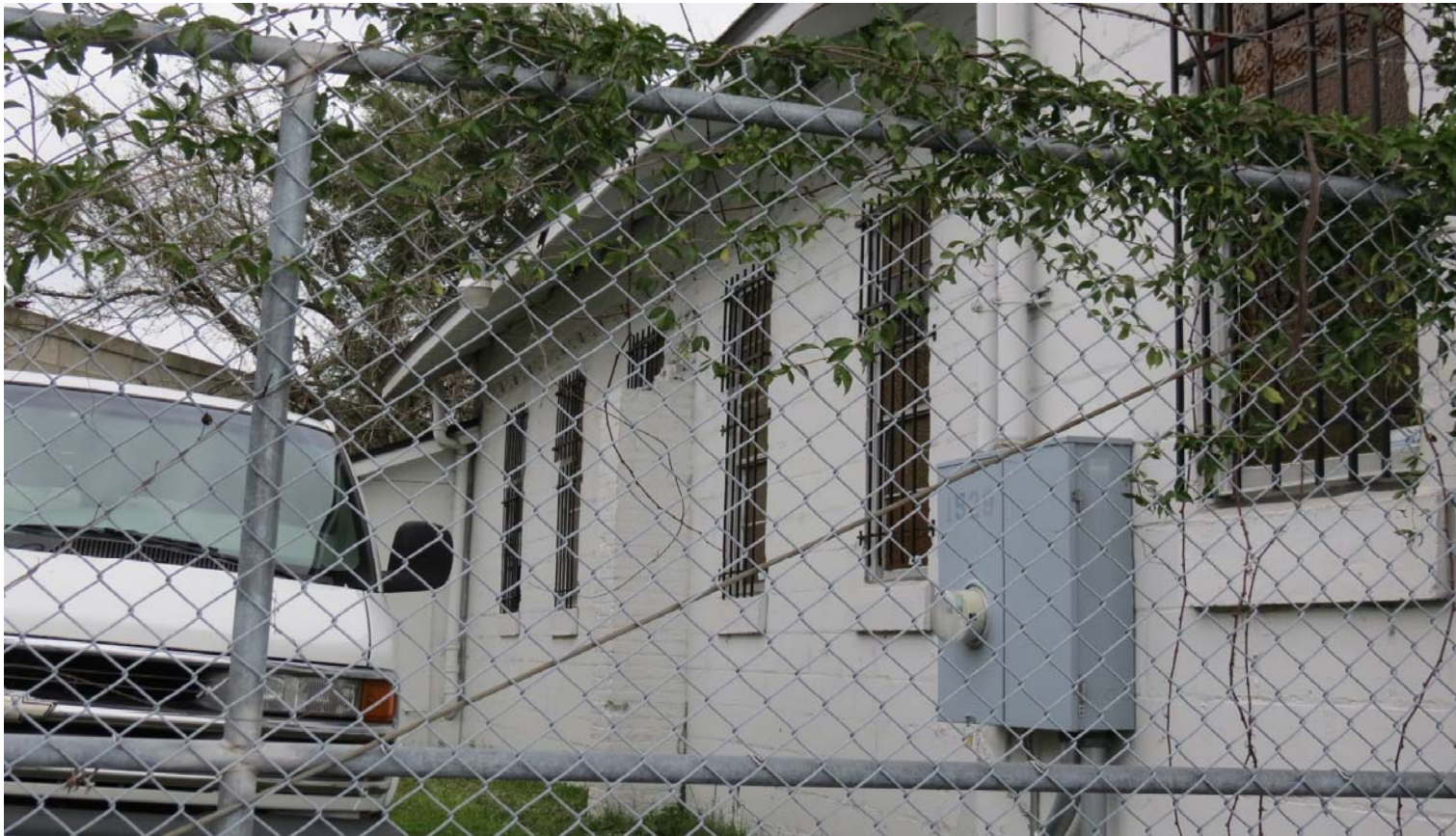
LM-19-01 ALLEN CHAPEL A.M.E. CHURCH 1529 SWAN STREET PHOTO # 30 JANUARY 4, 2019
