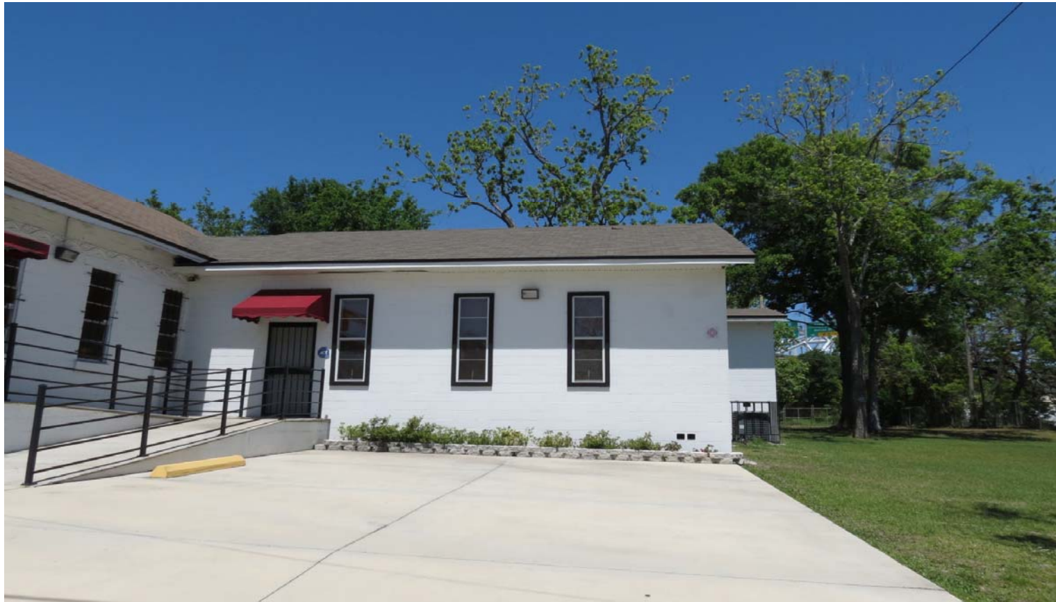
LM-19-01 ALLEN CHAPEL A.M.E. CHURCH 1529 SWAN STREET PHOTO # 25 APRIL 17, 2018
