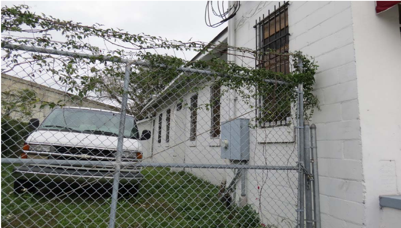
LM-19-01 ALLEN CHAPEL A.M.E. CHURCH 1529 SWAN STREET PHOTO # 29 JANUARY 4, 2019
