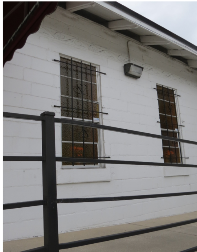
LM-19-01 ALLEN CHAPEL A.M.E. CHURCH 1529 SWAN STREET PHOTO # 23 JANUARY 4, 2019
