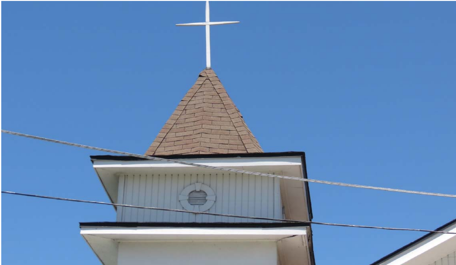
LM-19-01 ALLEN CHAPEL A.M.E. CHURCH 1529 SWAN STREET PHOTO # 13 APRIL 17, 2018
