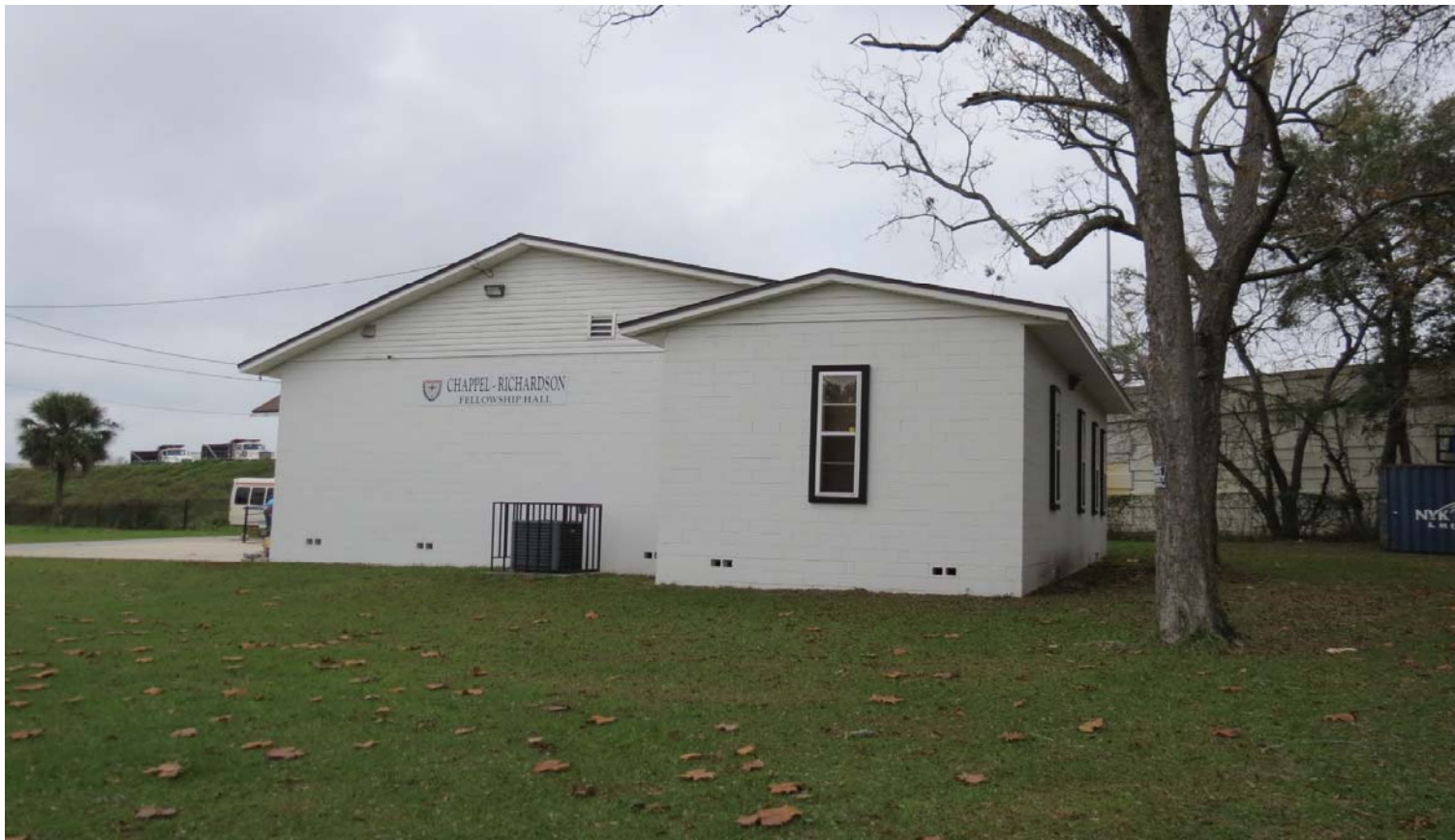
LM-19-01 ALLEN CHAPEL A.M.E. CHURCH 1529 SWAN STREET PHOTO # 28 JANUARY 4, 2019
