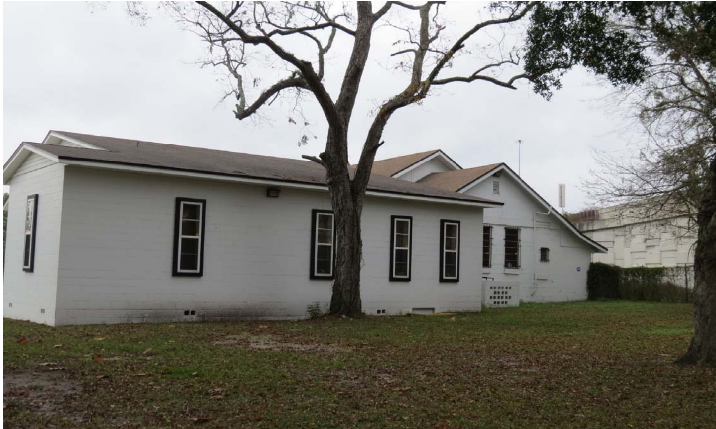
LM-19-01 ALLEN CHAPEL A.M.E. CHURCH 1529 SWAN STREET PHOTO # 37 JANUARY 4, 2019
