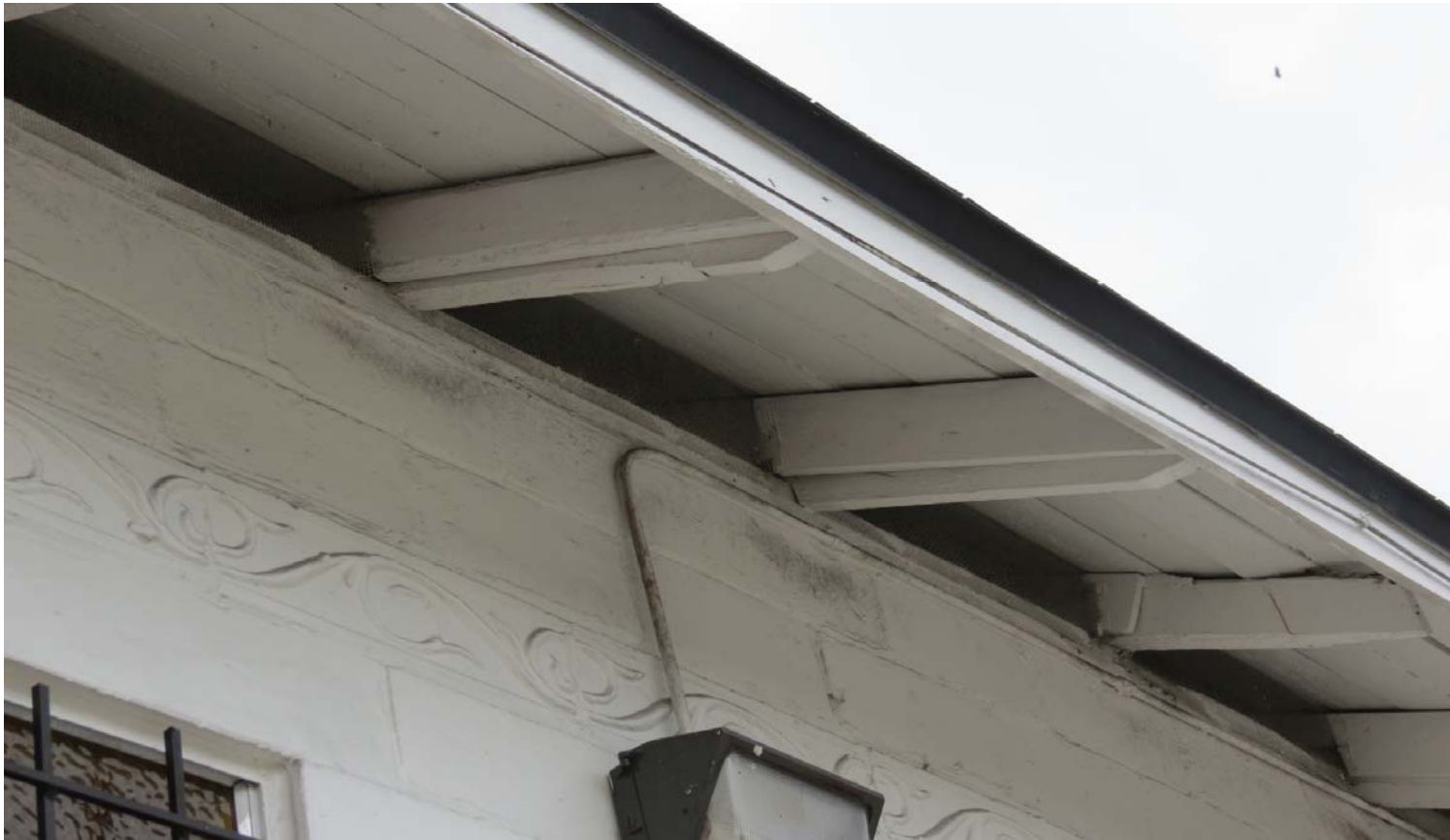
LM-19-01 ALLEN CHAPEL A.M.E. CHURCH 1529 SWAN STREET PHOTO # 34 JANUARY 4, 2019
