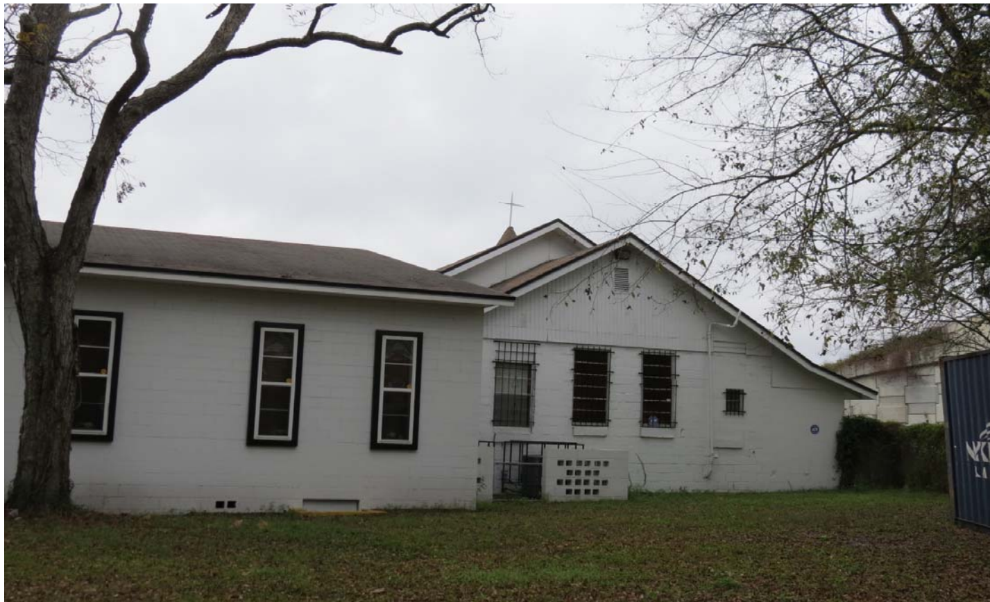
LM-19-01 ALLEN CHAPEL A.M.E. CHURCH 1529 SWAN STREET PHOTO # 39 JANUARY 4, 2019
