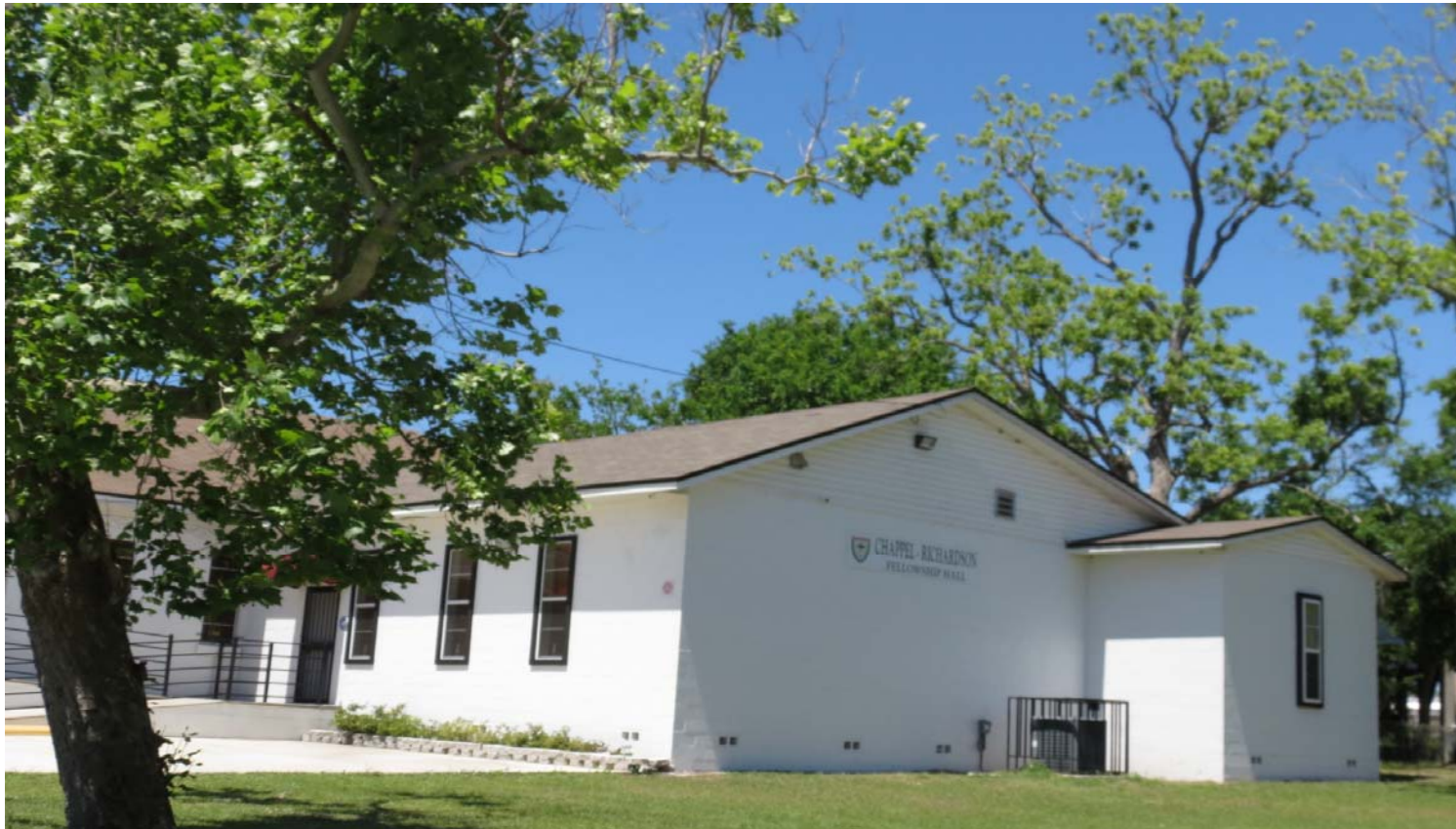
LM-19-01 ALLEN CHAPEL A.M.E. CHURCH 1529 SWAN STREET PHOTO # 26 APRIL 17. 2018
