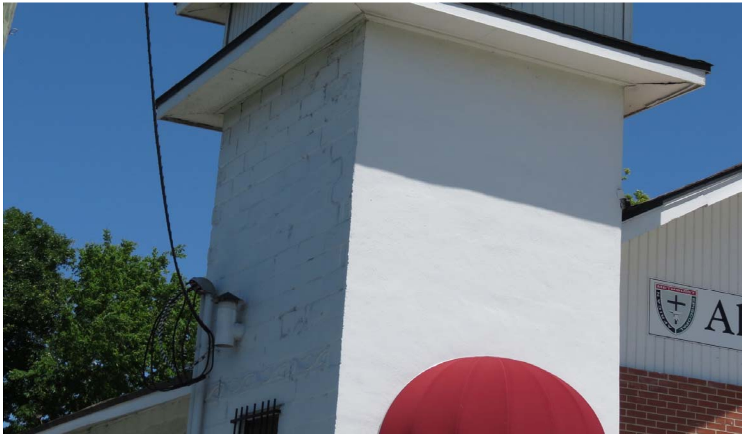
LM-19-01 ALLEN CHAPEL A.M.E. CHURCH 1529 SWAN STREET PHOTO # 12 APRIL 17, 2018
