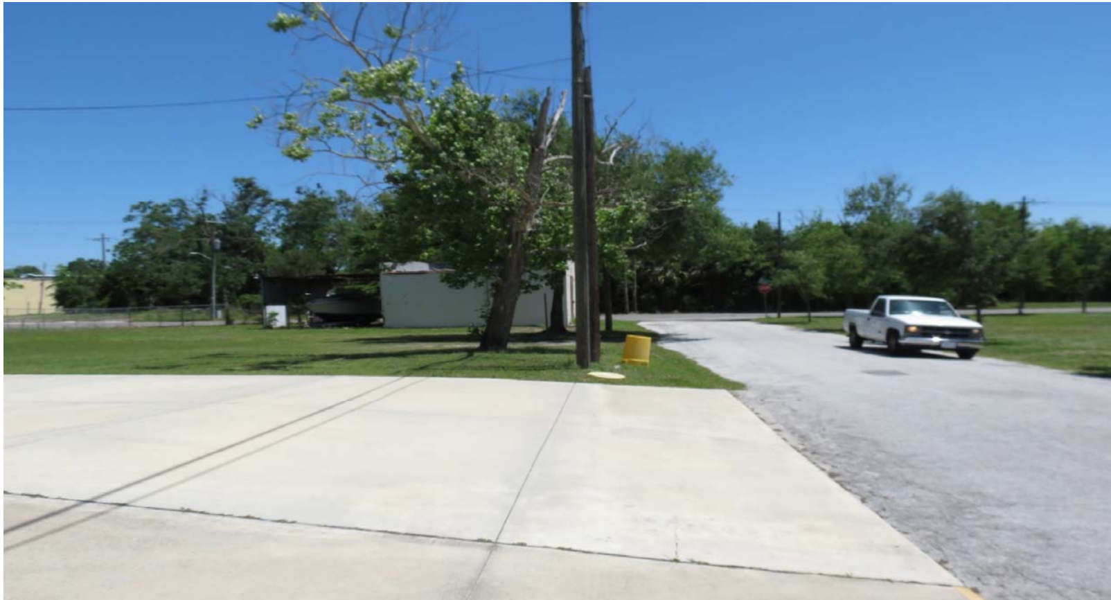
LM-19-01 ALLEN CHAPEL A.M.E. CHURCH 1529 SWAN STREET PHOTO # 6 APRIL 17, 2018
