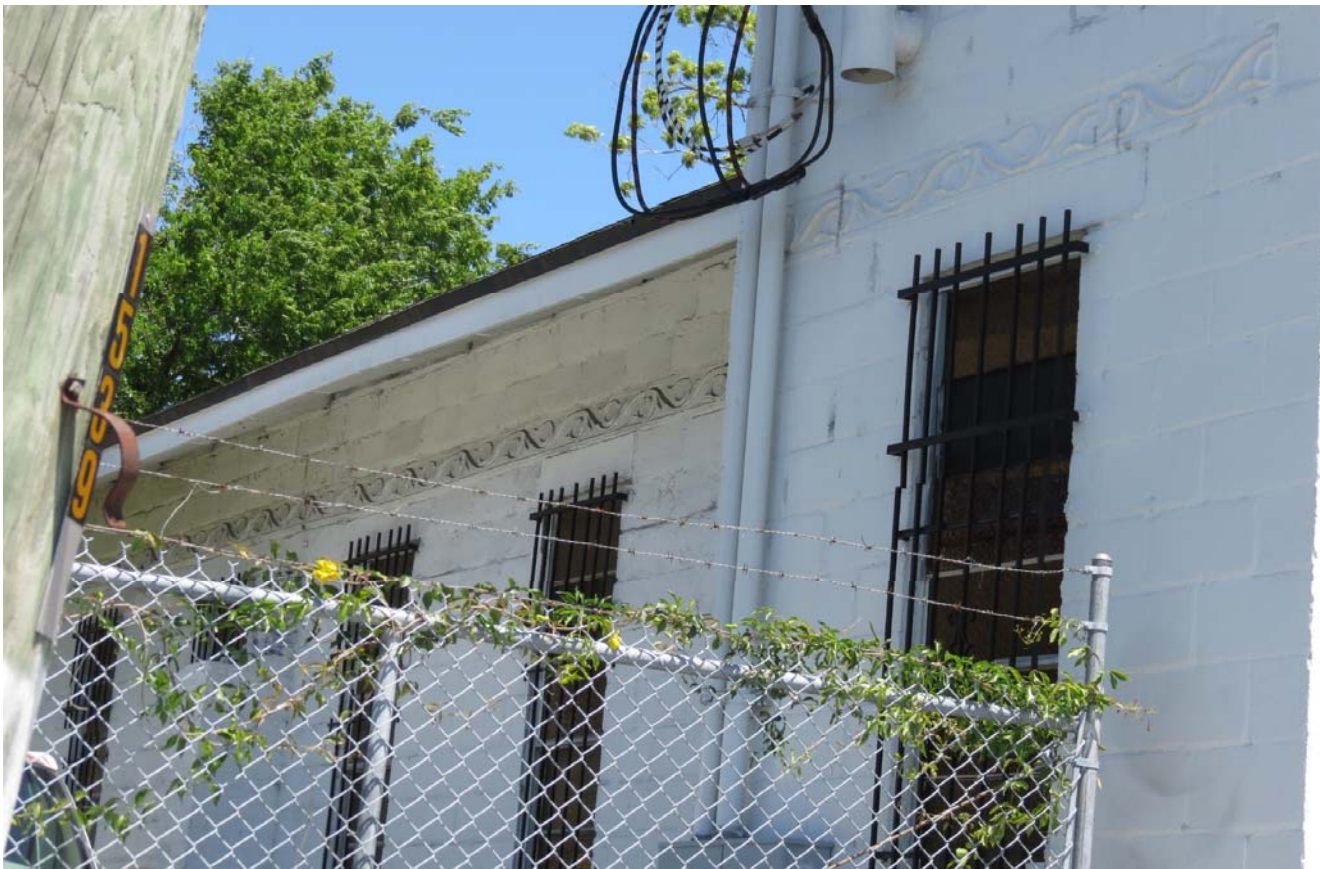
LM-19-01 ALLEN CHAPEL A.M.E. CHURCH 1529 SWAN STREET PHOTO # 32 APRIL 17, 2018
